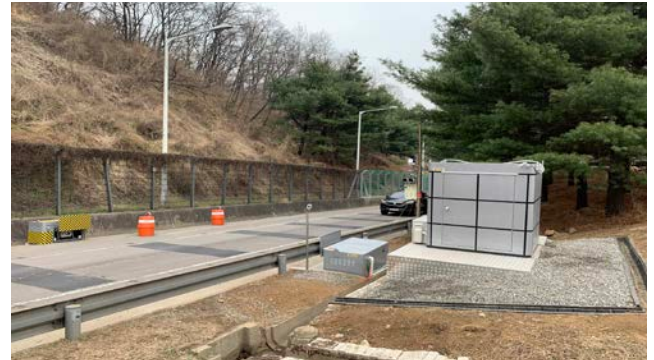
Unmanned fixed RSD at Naegok IC
